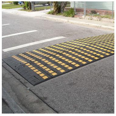
Slow vehicles to 10-20 mph, can be asphalt or rubber, Disadvantage: Also slow emergency vehicles.
