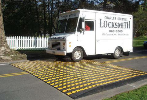
Slow vehicles to 20-25 mph. Advantage: Less aggressive, smoother to pass over than speed humps, do not slow emergency vehicles as much as humps.
