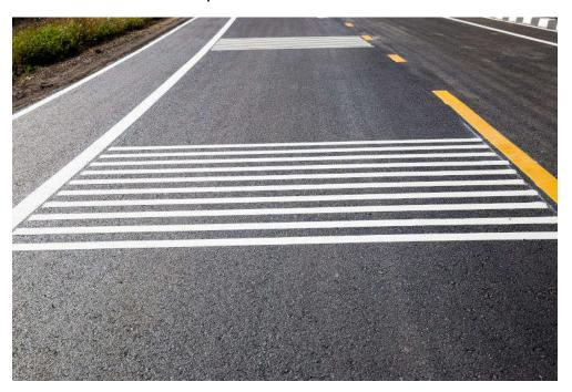
Low cost method of calming. Disadvantage: Only reduces speeds by 2-8 mph.
